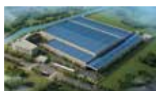
★ Jiangsu Forever Electro-Hydraulic Servo Production Base Wuxi (East & Middle China)
